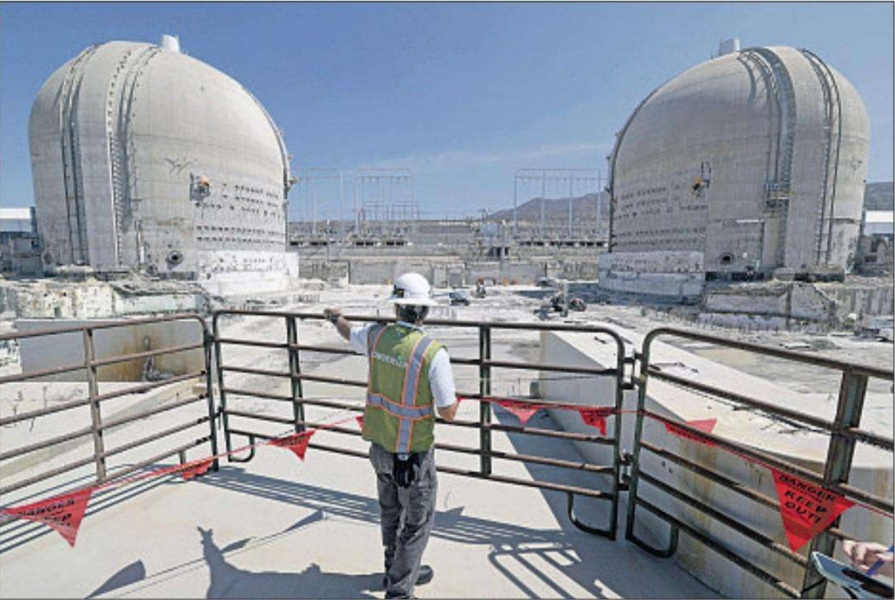
THE SHUTTERED plant near San Clemente is still home to 3.6 million pounds of high-level nuclear waste.
